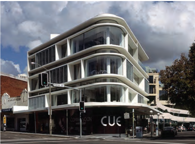
Commercial/ Retail Building, Double Bay
